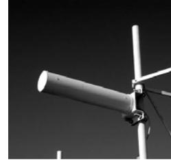
useful for very long range broadcast to fixed targets. The CTI 5636 14dBi Yagi Antenna (pictured right) is a very powerful, highly directional antenna, and is capable of significant range when installed correctly.
